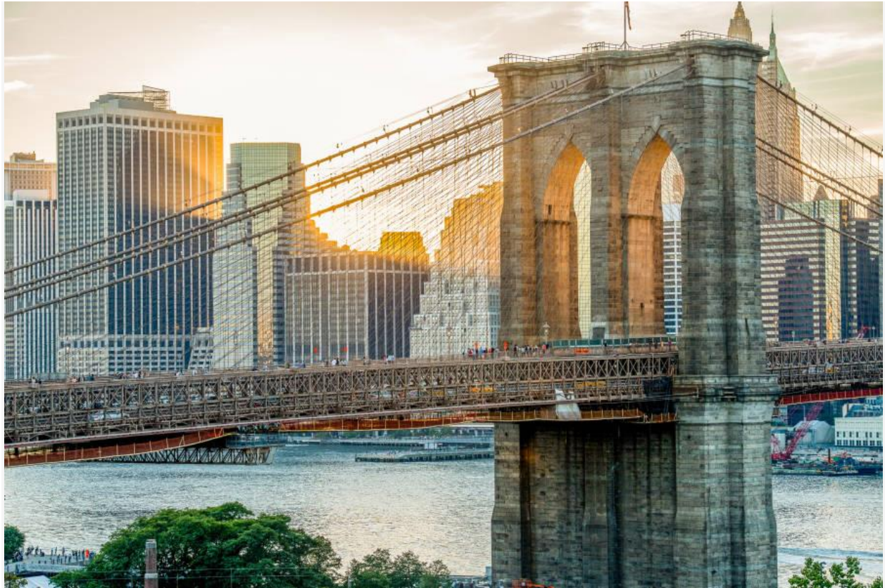
Brooklyn Bridge. Photo: Julianne Schaer
