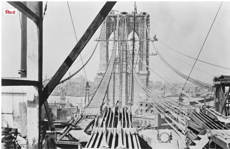
Cables are put in place on the Brooklyn Bridge during its construction, circa 1875. The bridge was designed with four main cables , which descend from the tops of the suspension towers and help support the deck.
