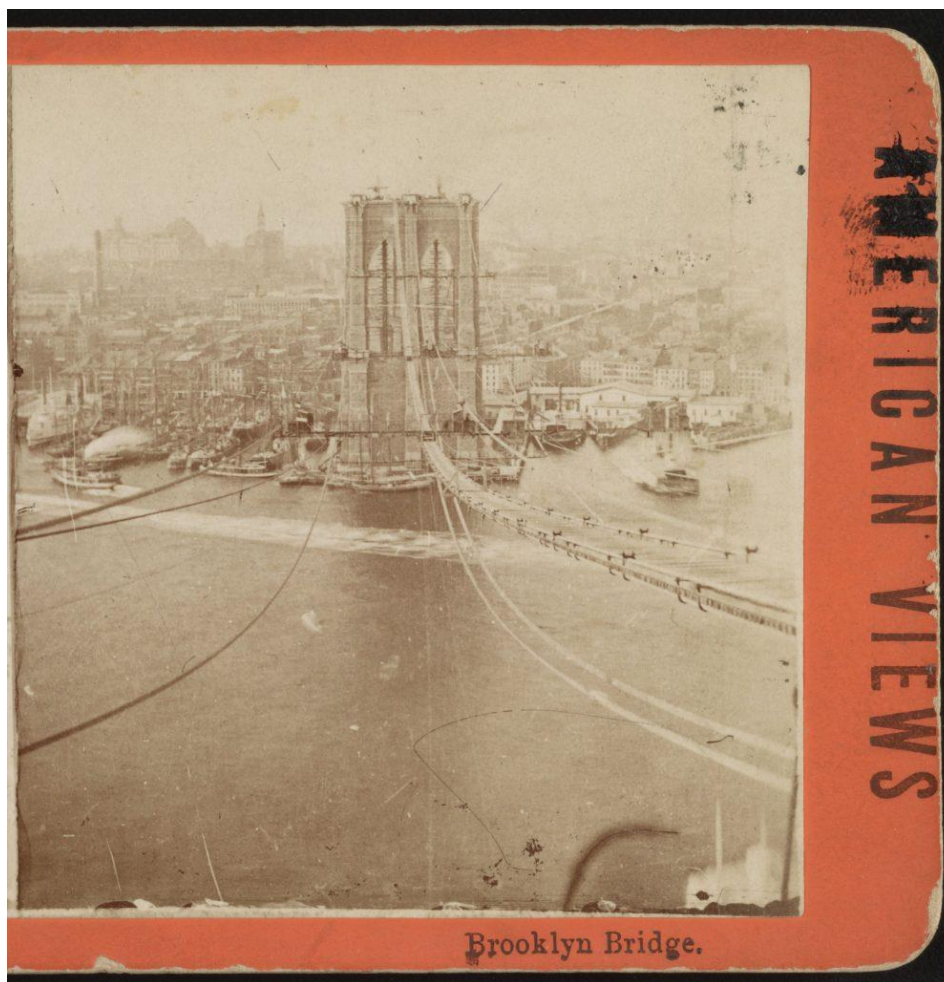
Brooklyn Bridge under construction, ca. 1873-1880. Stereocard. Library of Congress, Prints and Photographs Division.
