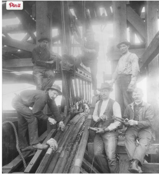
Workmen cutting and tying tension cables, circa 1882. Each of the bridge's four main cables is made of 19 separate strands, each of which has 278 separate wires.
